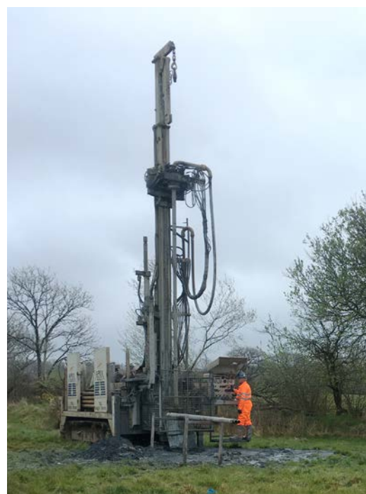
Sinking a borehole at Southern Roots Organics, Pembrokeshire
