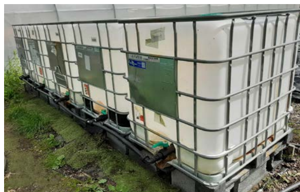
Pallet-mounted IBC's for rainwater storage, collected from a polytunnel
