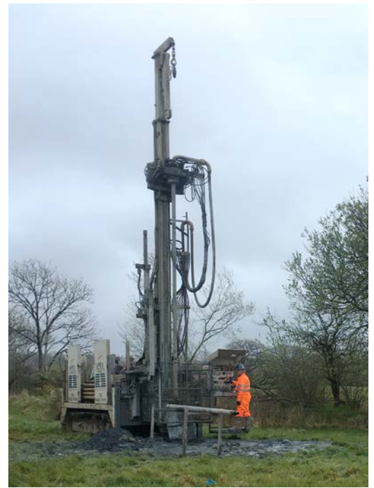
Sinking a borehole at Southern Roots Organics, Pembrokeshire
